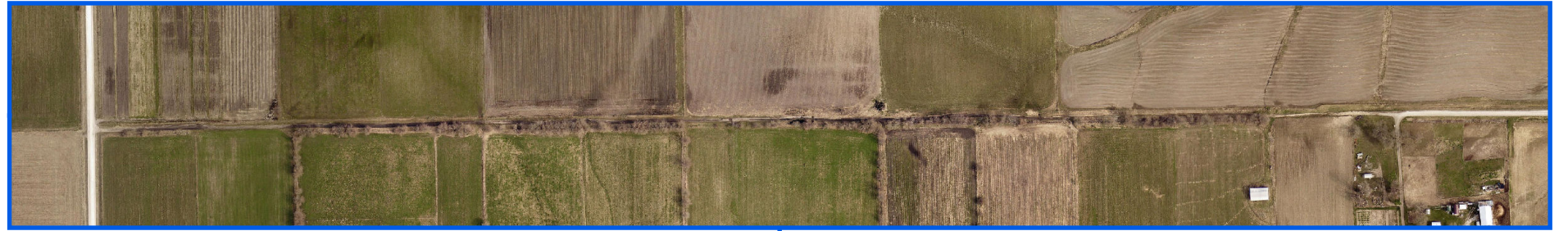
2021 Aerial Photo showing condition of road
